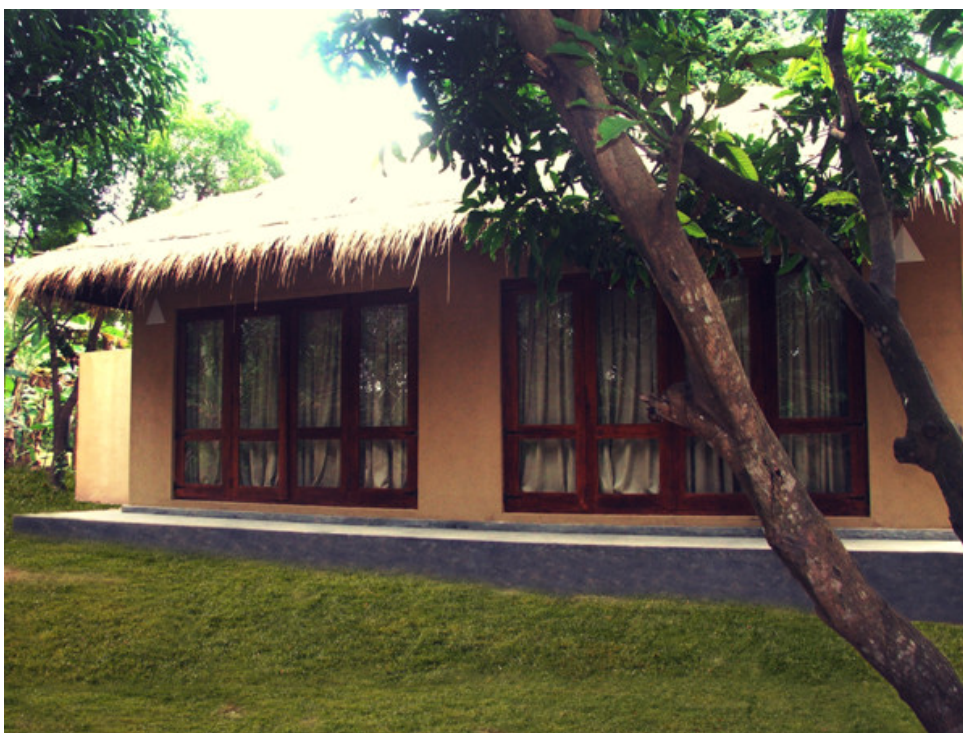
River Facing Cottage At Wild Escape
