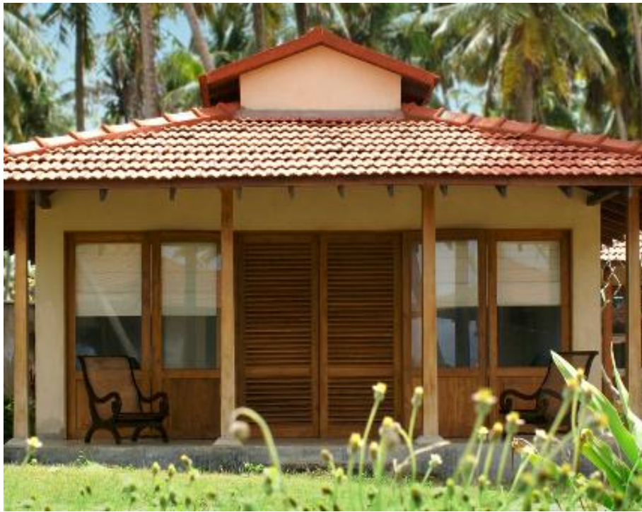
Front View Of Garden Villa
