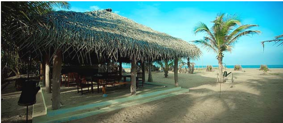
Dining Pavilion Exterior
